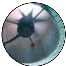
Detalle Chimenea Chimney detail
